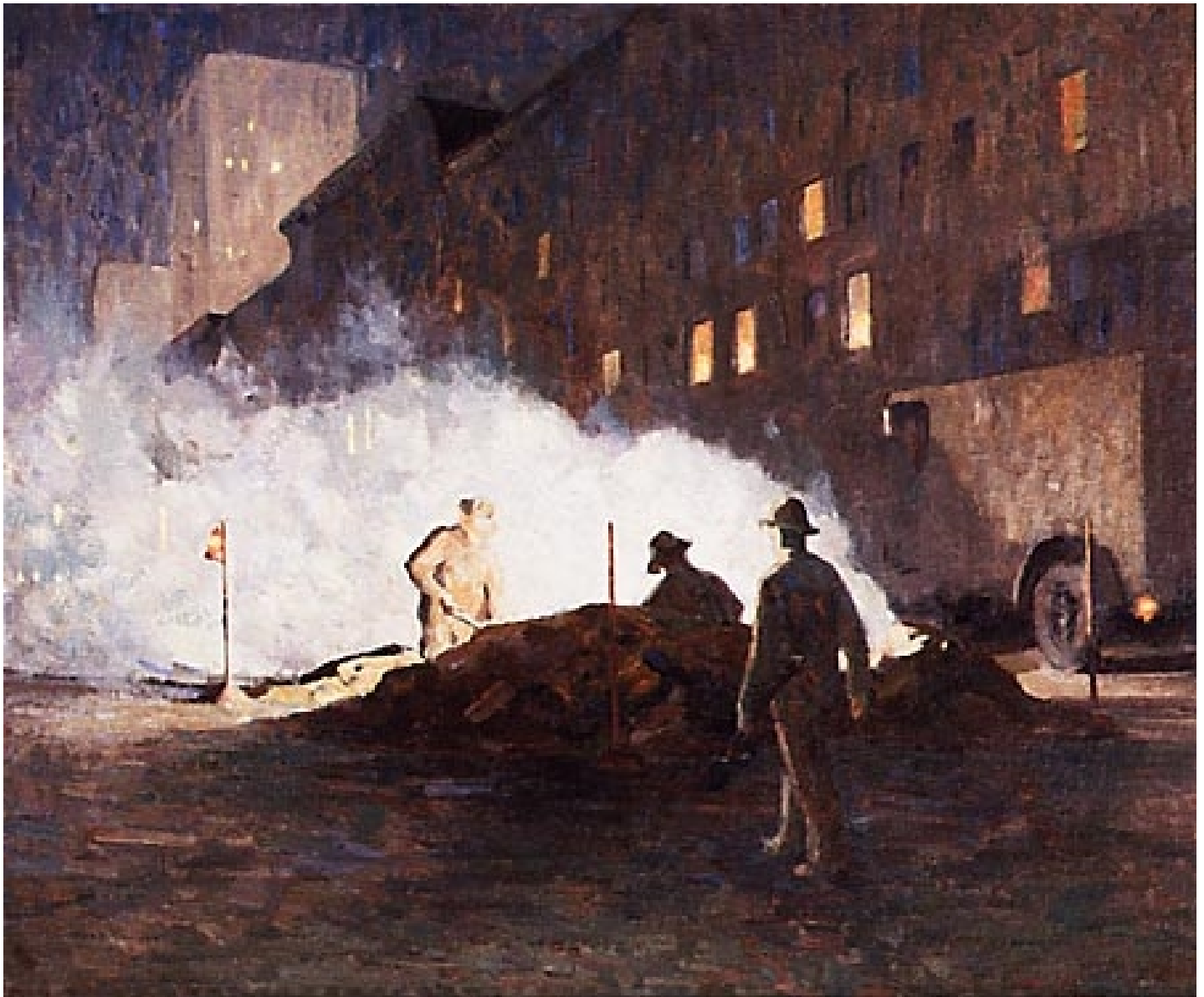
Dines Carlsen, Steam Pipe Repair Crew oil on canvas, 25 x 30 in. (63.5 x 76.2 cm) DC190401
